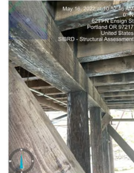
Photo 03: MC Pier Substructure Marine Consortium Pier Pile Cap Typical condition of pile caps Moata ID: Not Applicable
