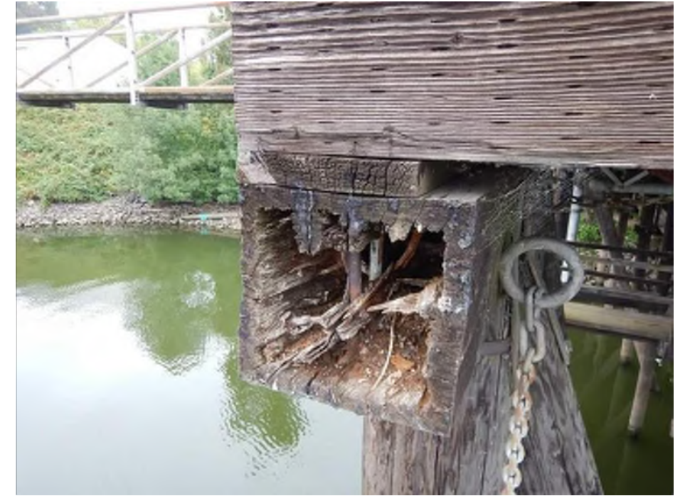
Photo 03: U.S. Navy Pier Substructure Timber pile cap with severe end grain fungal decay Source: AME 2019 Report
