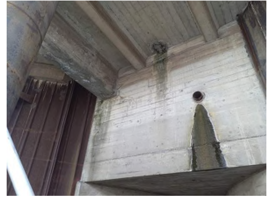
Photo 03: Quay Wall Substructure Concrete Pile Cap between Sheet Piles F-F and E-E Closed spall on the bottom of the concrete pile cap Moata ID: 74941
