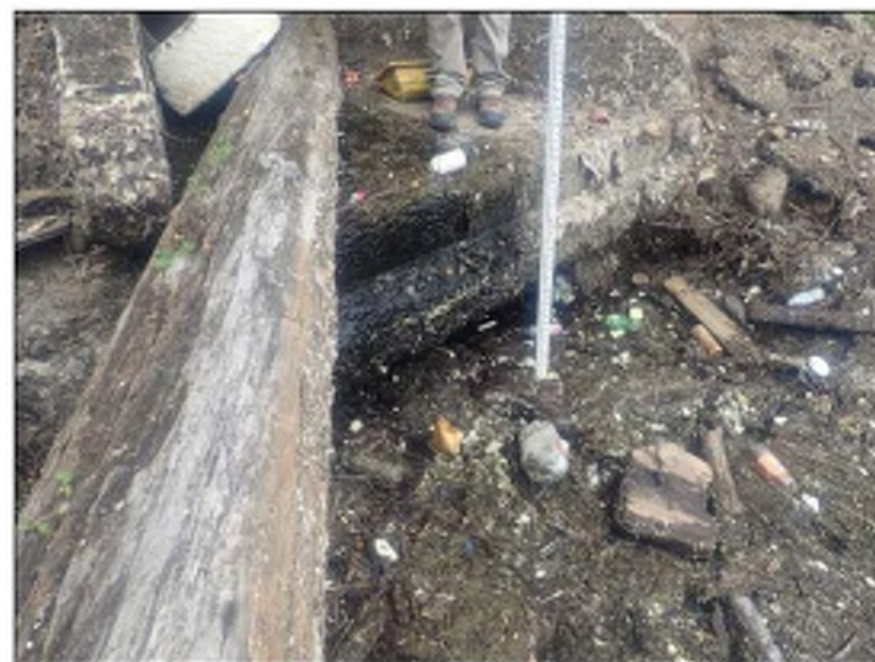
Photo 05: City Stormwater Outfall S2 Base Undermining at outfall
