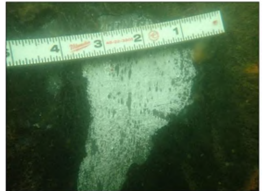
Photo 03: Pier C Substructure Typical cleaned surface of steel piles below waterline
