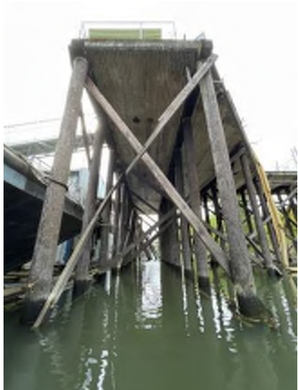
Photo 03: Lay Berth 307 Substructure Cross-Bracing at Bent 1 Broken cross-bracing Moata ID: 75042
