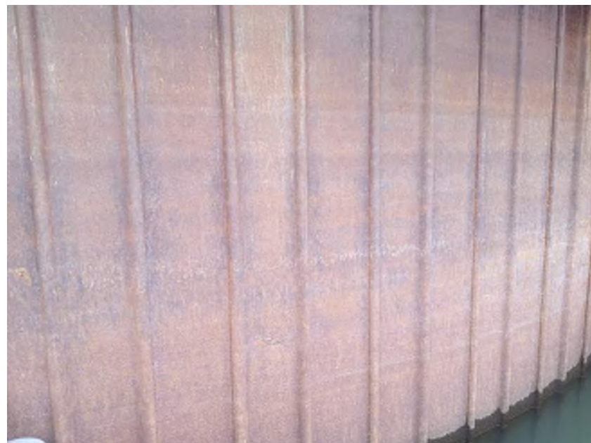
Photo 04: Quay Wall Substructure Sheet Pile C-C Typical condition of sheet piles above water Moata ID: Not Applicable
