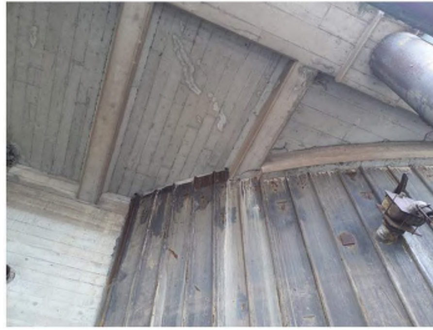
Photo 02: Quay Wall Substructure Concrete Pile Cap between Sheet Piles F-F and E-E Crack on the bottom of the concrete beam Moata ID: 74941
