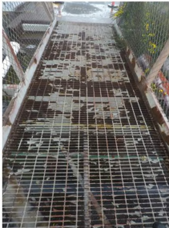
Photo 03: East Pier Superstructure Steel Grate Between Pier End to Bent 1 Typical condition of steel grate (minor corrosion) Moata ID: Not Applicable
