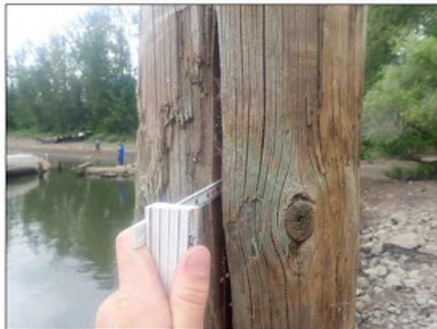
Photo 03: Swan Island Boat Ramp Piles Typical checking on timber piles
