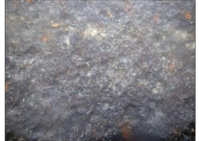
Photo 03: Quay Wall Substructure Typical pitting on steel sheet pile cells at waterline
