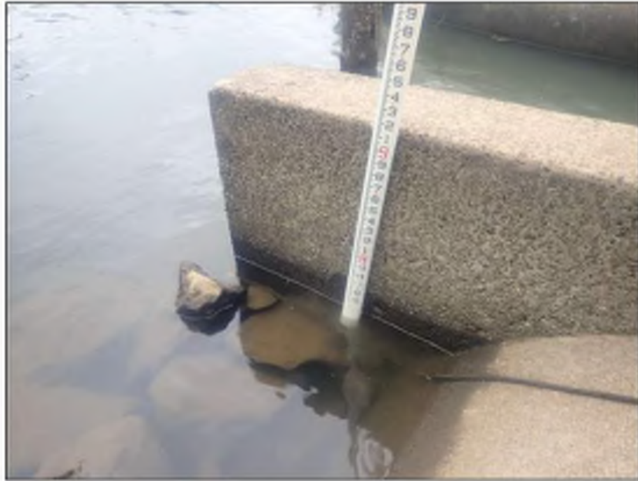
Photo 01: City Stormwater Outfall M3 Wingwalls Typical condition of concrete at waterline
