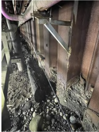
Photo 14: Lagoon Wharf Substructure Steel Sheet Piles between Bents 59 and 67 Corroded steel sheet piles Moata ID: Not Applicable
