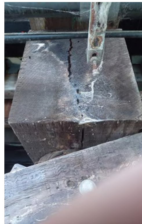
Photo 08: Lagoon Wharf Substructure Adjacent to Bent 16 Split on the pile cap Moata ID: 73784
