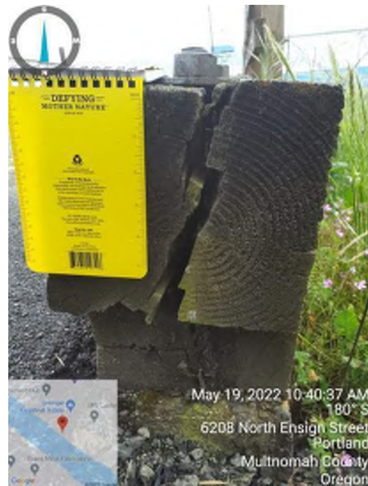
Photo 01: Dredge Base Superstructure End of Bullrail Split on the bullrail Moata ID: 74436
