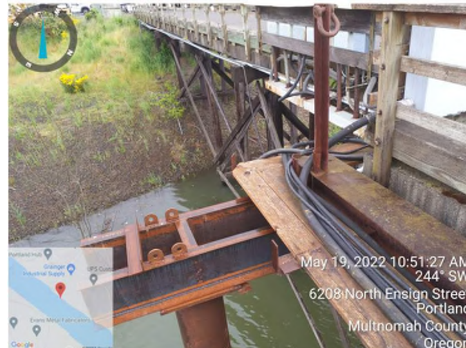
Photo 05: Dredge Base Substructure Pile Cap at Bents 5 Typical condition of pile cap Moata ID: Not Applicable
