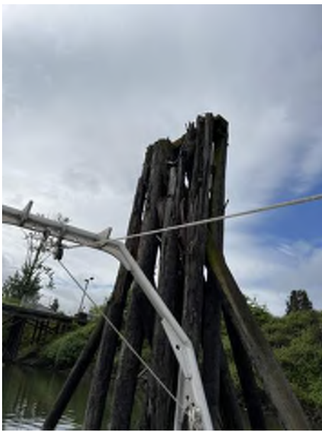
Photo 05: Lay Berth 307 Dolphin Dolphin D6 Broken piles Moata ID: 75063
