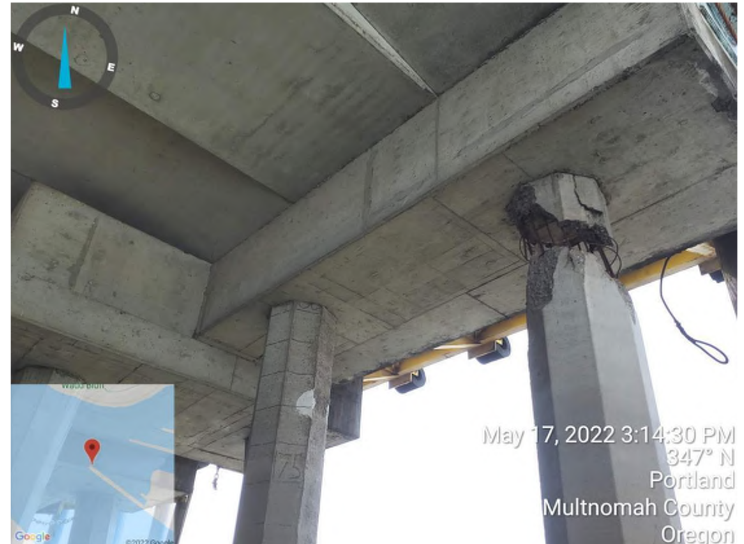
Photo 07: Pier D Substructure Pile K at Bent 1 Complete breakage at the top of Pile K Moata ID: Not Applicable
