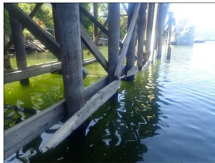
Photo 02: Lay Berth 308 Substructure Typical condition of walers at waterline
