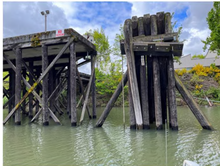
Photo 03: Lay Berth 308 Dolphin Dolphin D11 Broken piles at Dolphin D11 Moata ID: Not Applicable
