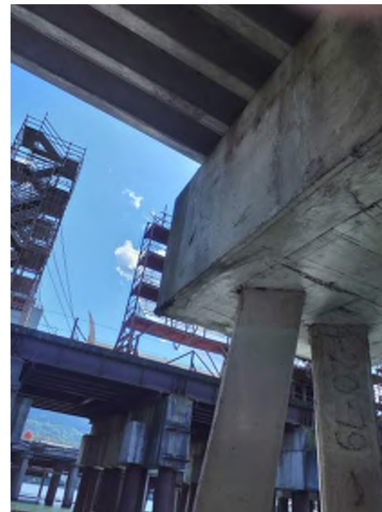
Photo 04: East Pier Superstructure Pile Cap between Bents 2 and 3 Concrete spall on the bottom of the pile cap Moata ID: 74982
