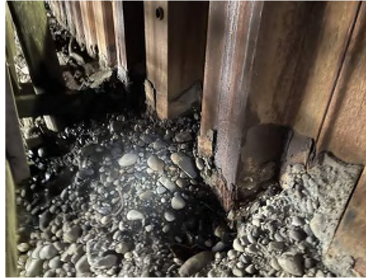
Photo 15: Lagoon Wharf Substructure Steel Sheet Piles between Bents 52 and 58 Typical condition of at bottom of steel sheet piles Moata ID: Not Applicable
