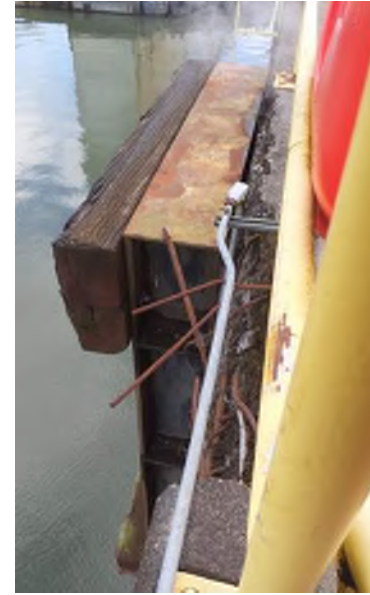
Photo 02: Pier C Superstructure Concrete Bullrail Between Bents 25 and 26 Concrete open spall exposing reinforcement Moata ID: 73679
