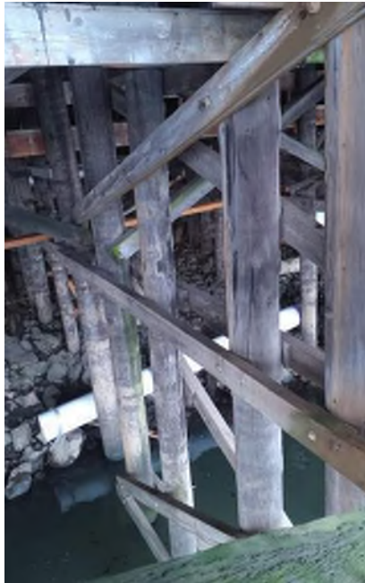
Photo 11: Lagoon Wharf Substructure Adjacent to Bent 13 Typical condition of the piles Moata ID: 73582
