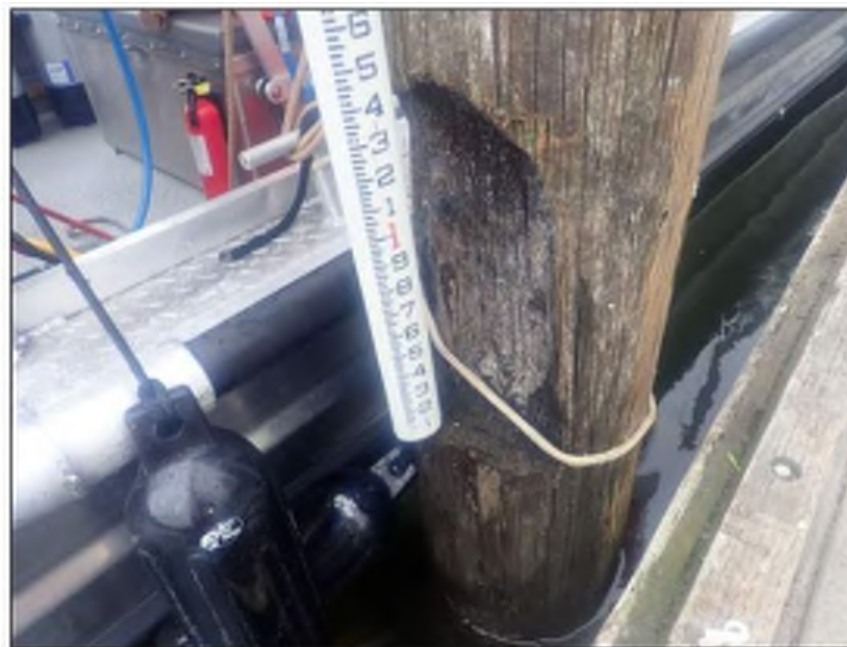
Photo 04: Swan Island Boat Ramp Piles Pile 5 Loss of section
