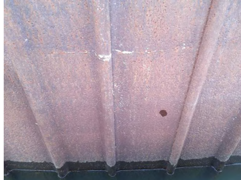
Photo 05: Quay Wall Substructure Sheet Pile C-C Typical condition of sheet piles above water Moata ID: Not Applicable
