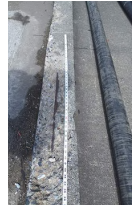
Photo 03: Pier D Superstructure Bullrail between Bents 22 and 23 Concrete spall exposing reinforcement Moata ID: 73720
