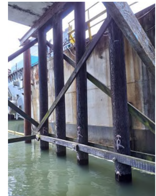
Photo 03: Dredge Base Substructure Piles at Bent 6 Typical condition of piles Moata ID: 74435
