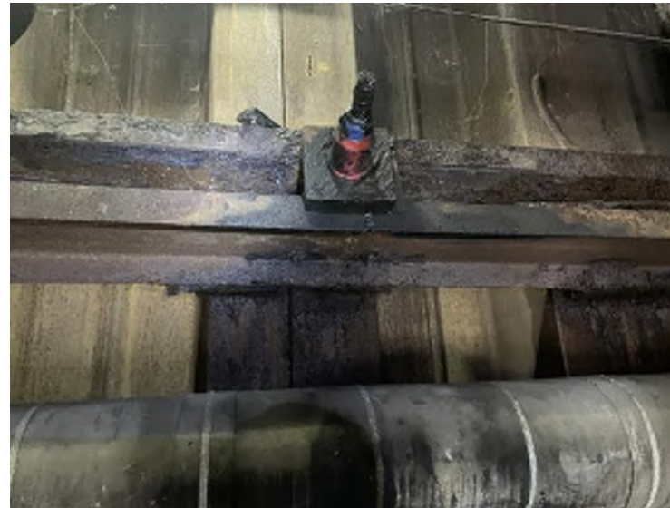
Photo 17: Lagoon Wharf Substructure Steel Sheet Piles between Bents 77 and 84 Corroded steel waler Moata ID: Not Applicable
