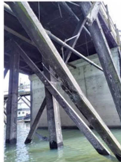
Photo 05: Berth 311 Trestle West Trestle Broken cross-bracing Moata ID: Not Applicable
