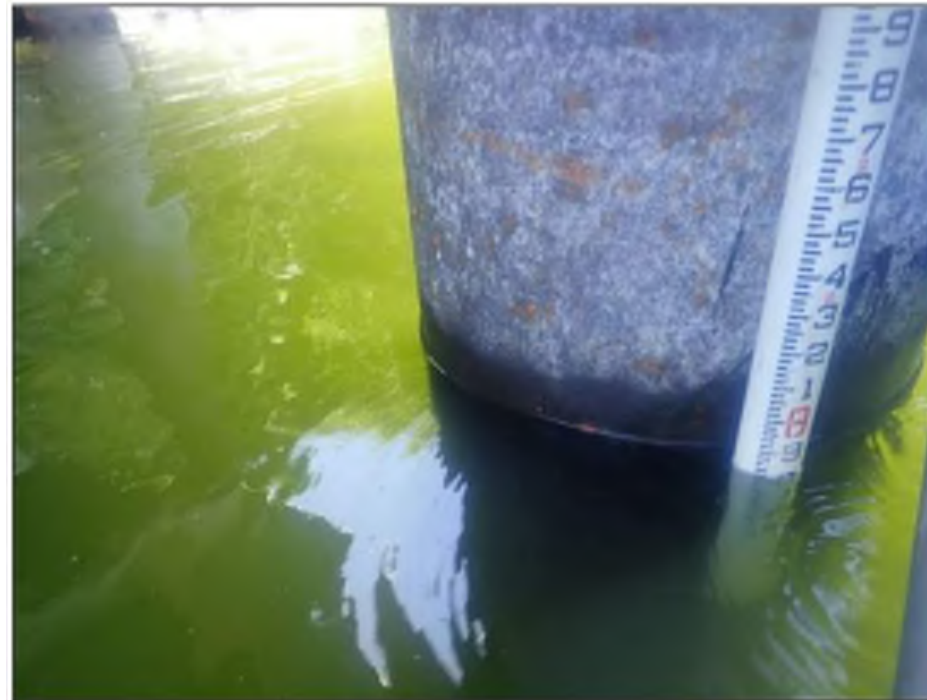
Photo 02: Wind Tunnel Substructure Typical condition of steel piles at waterline
