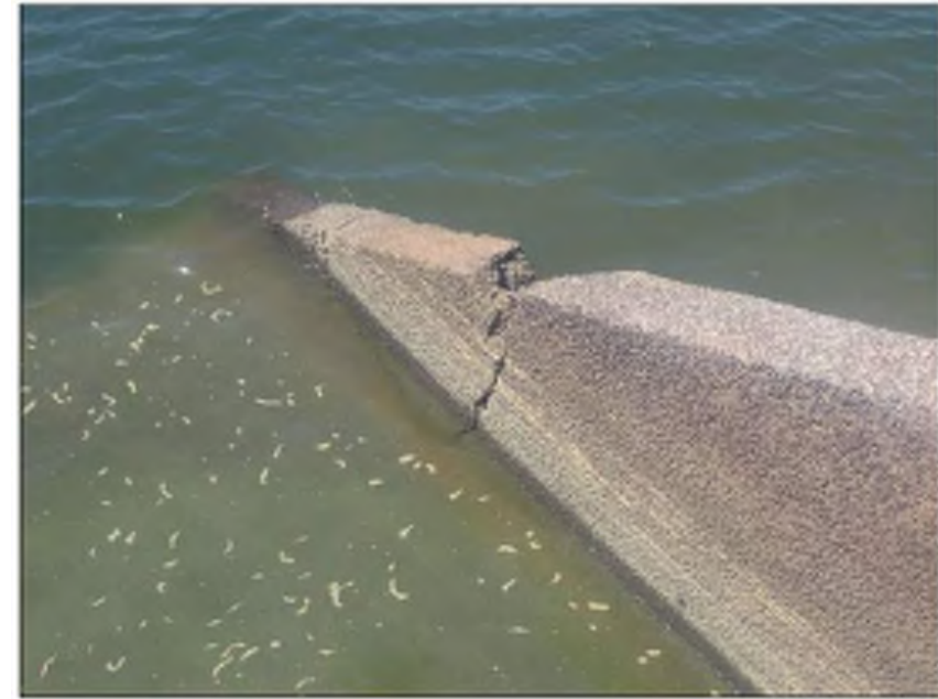
Photo 02: City Stormwater Outfall M1 Wingwalls West Wingwall Fractured west wingwall
