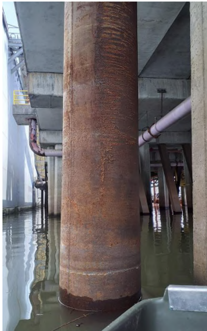
Photo 06: Pier D Substructure Pile K at Bent 21 Typical condition of steel piles above water Moata ID: 74360
