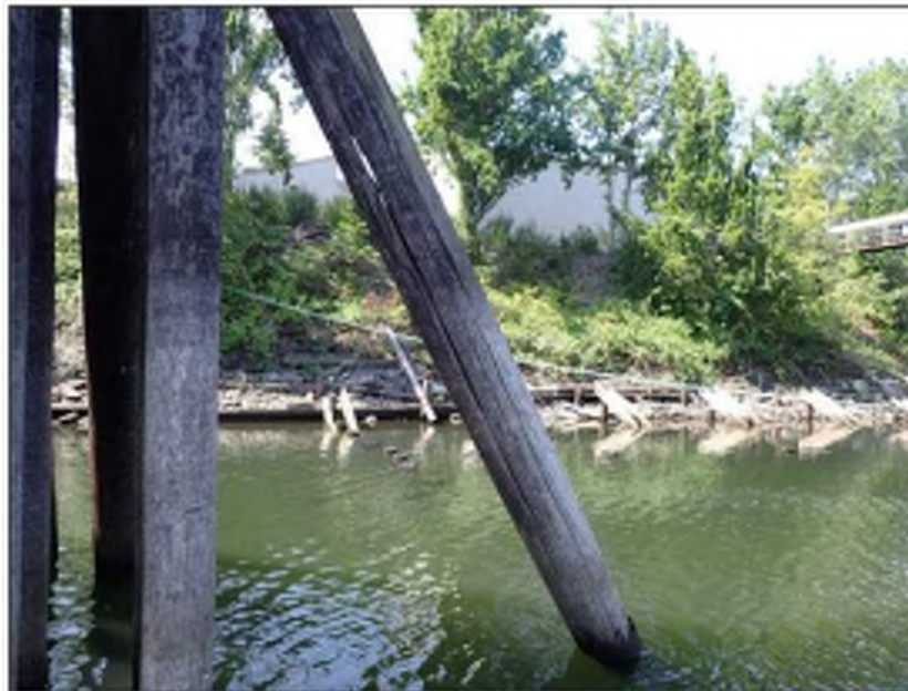
Photo 05: Lay Berth 308 Dolphins Dolphin D11, Pile 11 Timber pile decay
