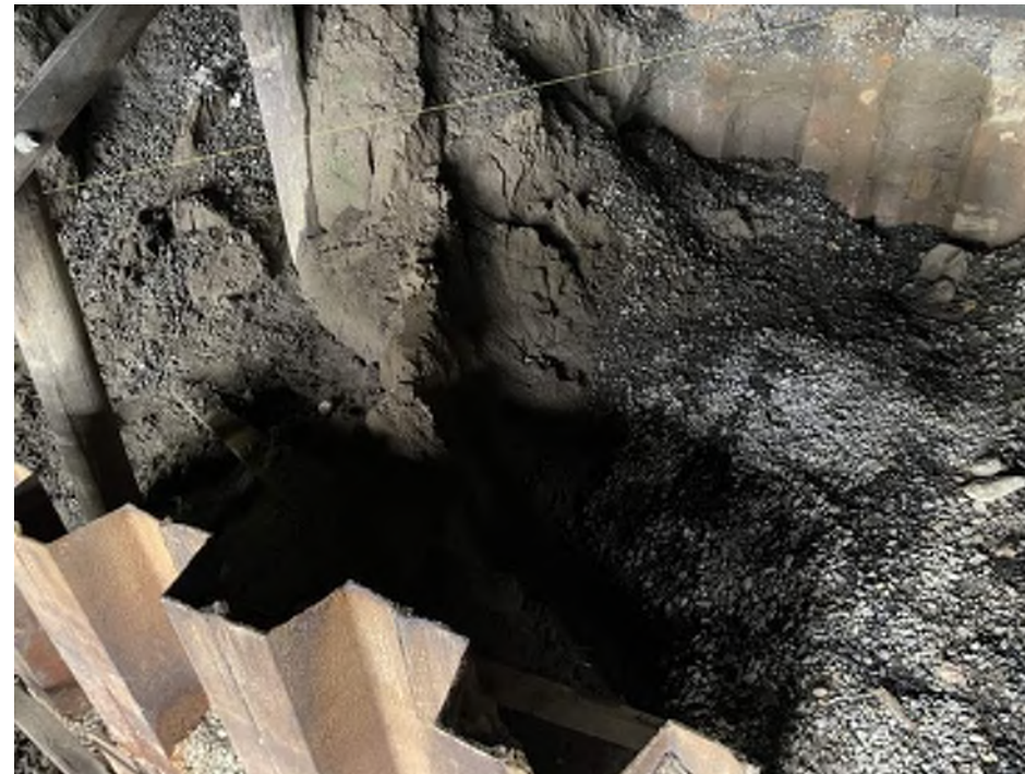
Photo 04: City Stormwater Outfall S1 Embankment erosion behind and adjacent to headwall
