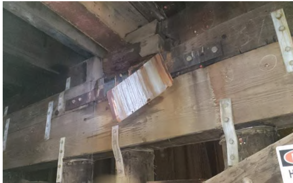
Photo 05: Lagoon Wharf Substructure Adjacent to Bent 3 Bearing plate severely corroded Moata ID: 73587
