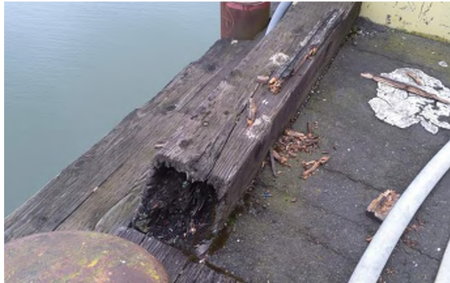
Photo 01: Lagoon Wharf Superstructure Timber Bullrail between Bents 133 and 134 Loss of section on bullrail Moata ID: 73540
