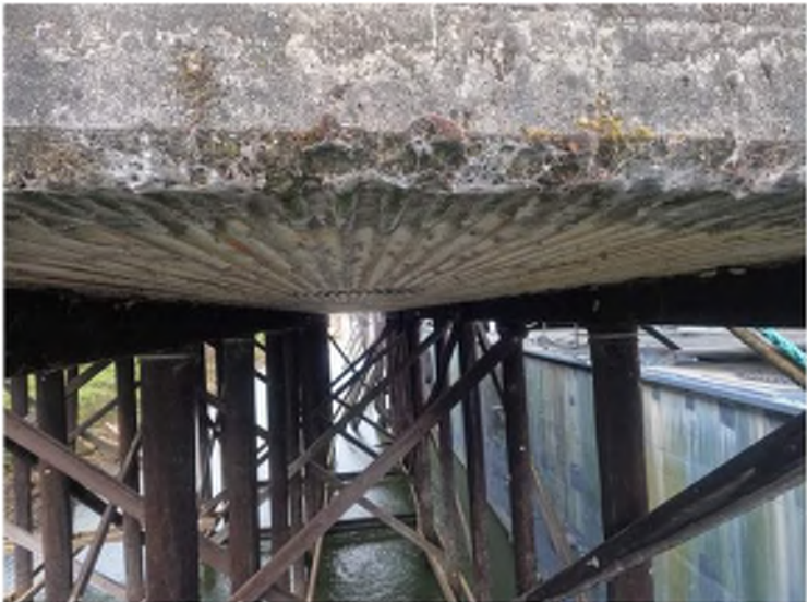
Photo 02: Lay Berth 307 Superstructure Underside of Concrete Deck Overview Typical condition of underside of concrete deck Moata ID: Not Applicable
