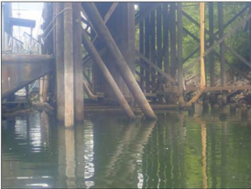
Photo 01: Lay Berths 306 & 307 Substructure Typical substructure configuration
