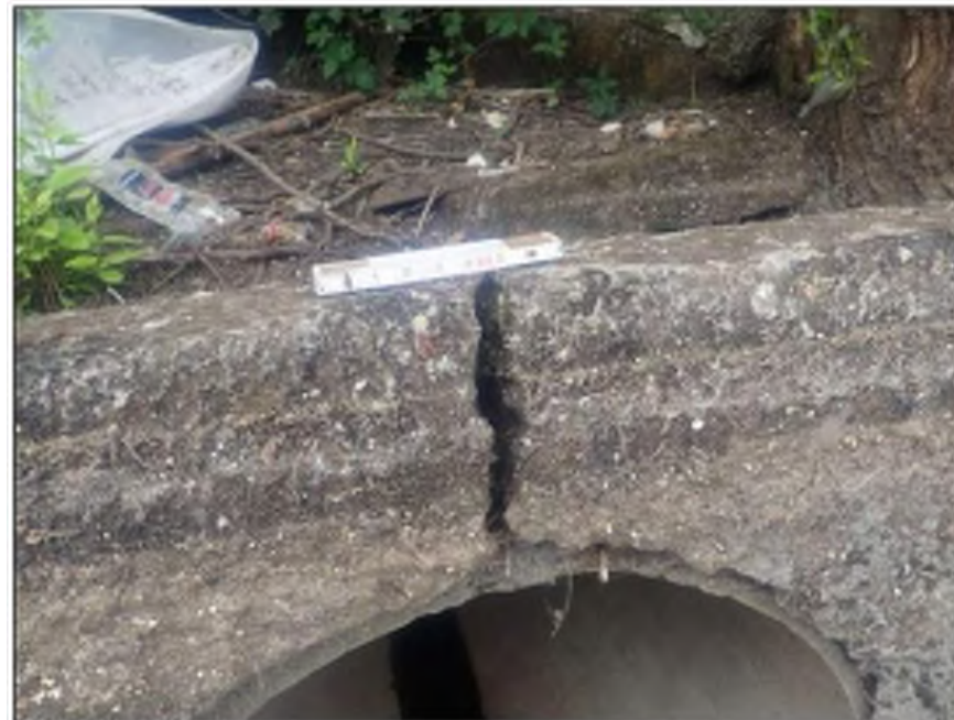
Photo 02: City Stormwater Outfall S2 Headwall Crack in top of head wall
