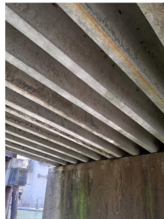
Photo 04: West Pier Substructure Concrete Girders between Bent 3 to Bent 4 Concrete spalls exposing reinforcement due to corrosion Moata ID: 74980
