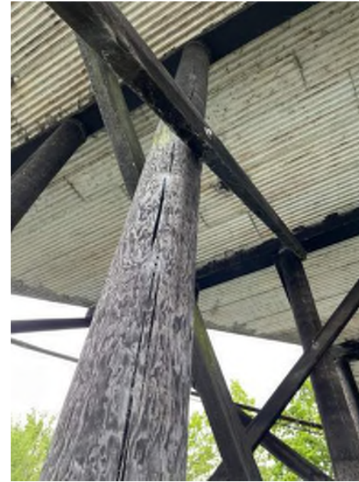
Photo 02: Lay Berth 308 Substructure Bent 7 Pile B Typical condition of piles Moata ID: 75057
