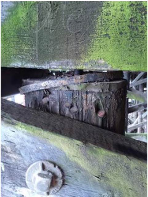
Photo 12: Lagoon Wharf Substructure Adjacent to Bent 129 Pile fully non-bearing Moata ID: 74274
