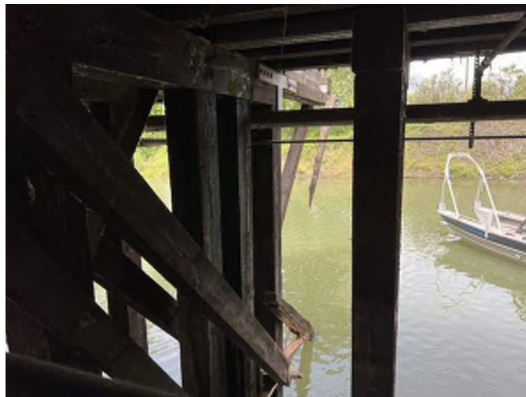
Photo 10: Berth 311 Main Pier Cross-Bracing at Bent 26 Broken cross-bracing Moata ID: 74410
