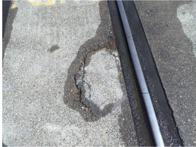
Photo 01: Pier C Superstructure Concrete Deck Between Bents 45 and 46 Concrete closed spall on the top of the deck Moata ID: 73677
