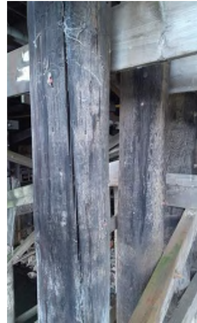
Photo 19: Lagoon Wharf Substructure Adjacent to Bent 17 Split on the timber pile Moata ID: 73579
