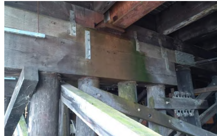
Photo 04: Lagoon Wharf Substructure Adjacent to Bent 3 Typical condition of pile caps Moata ID: 73586
