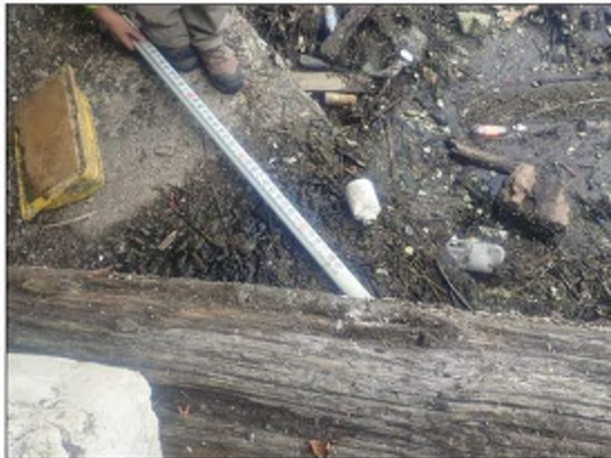
Photo 04: City Stormwater Outfall S2 Outfall Base Abrasion on outfall surface
