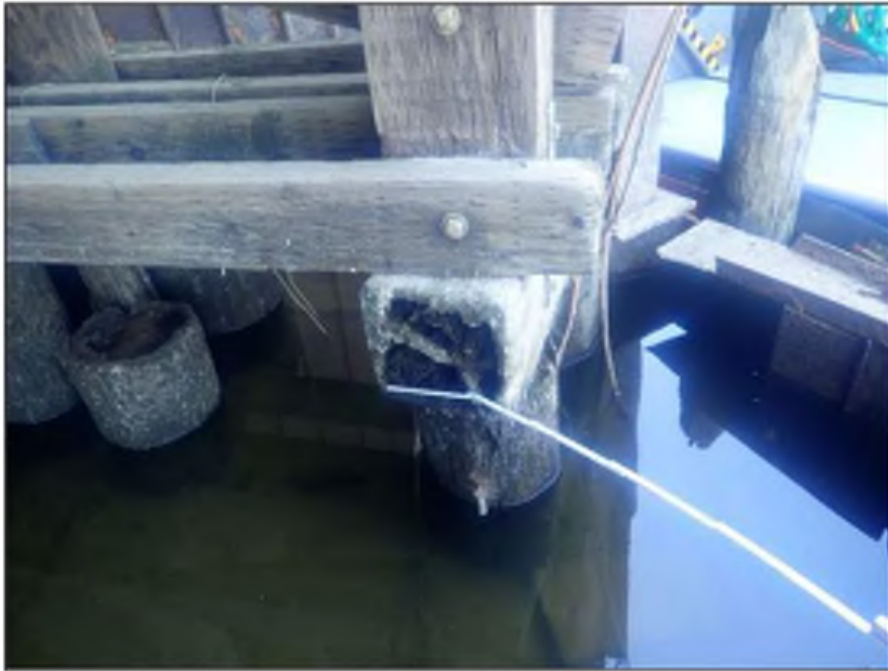
Photo 07: Lagoon Wharf Substructure Core decay in water support square piles at bent 0
