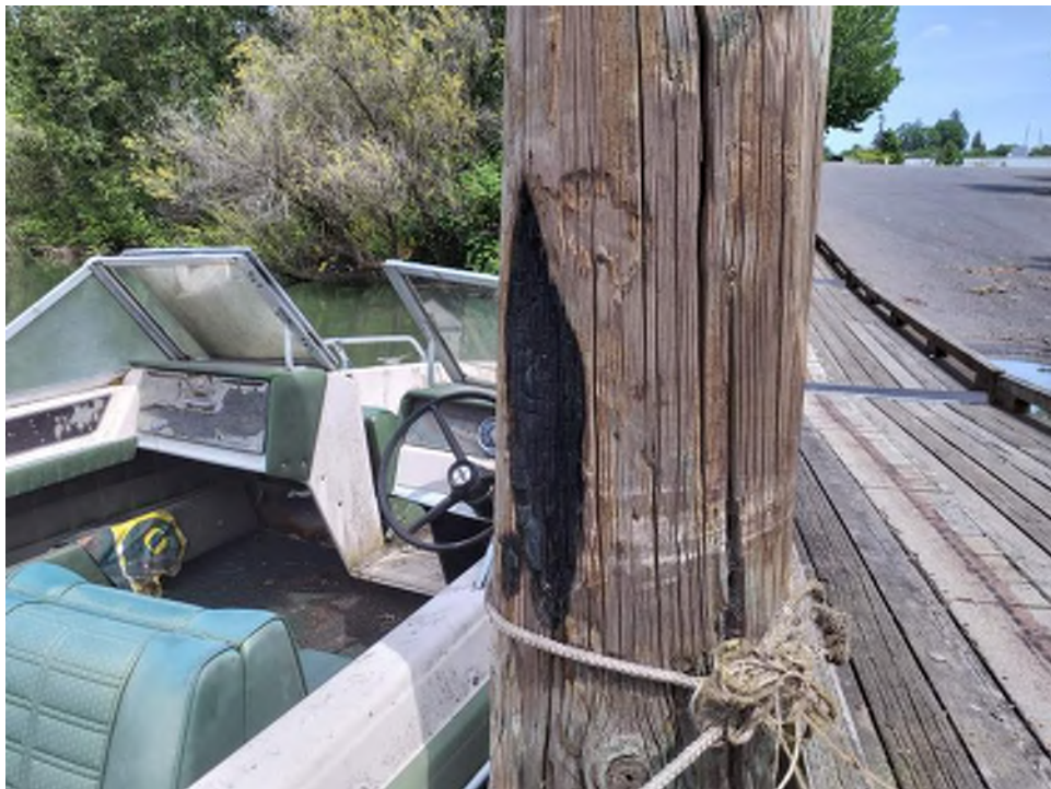
Photo 03: Swan Island Boat Ramp Piles Pile 3 Loss of section on pile Moata ID: 74345
