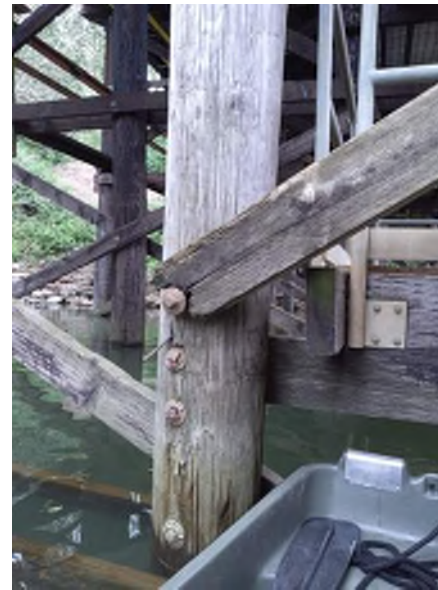
Photo 02: U.S. Coast Guard Dock and Pier Substructure Cross-bracing Between Piles D and F at Bent 9 Broken cross-bracing Moata ID: 74996
