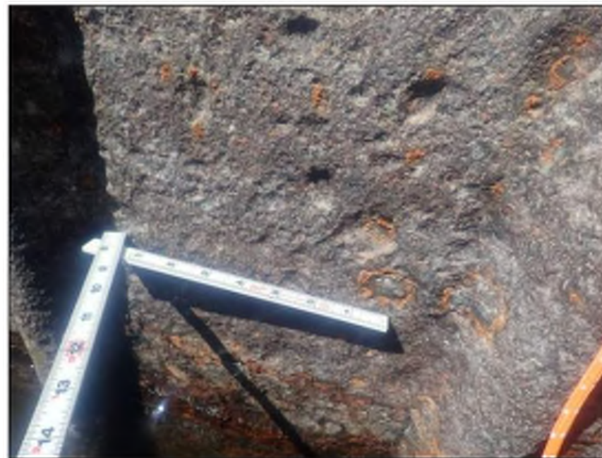
Photo 02: Pier A Substructure Typical pitting on sheet pile cells at waterline
