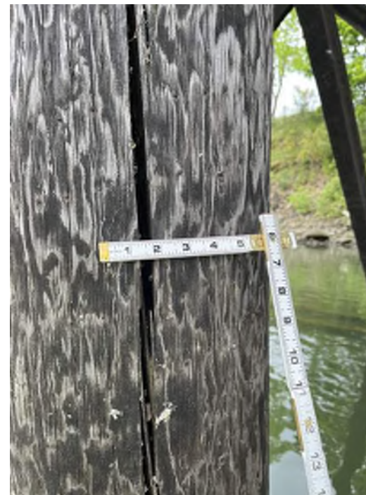
Photo 04: Lay Berth 308 Substructure Bent 7 Pile B Split on the timber pile Moata ID: 75057
