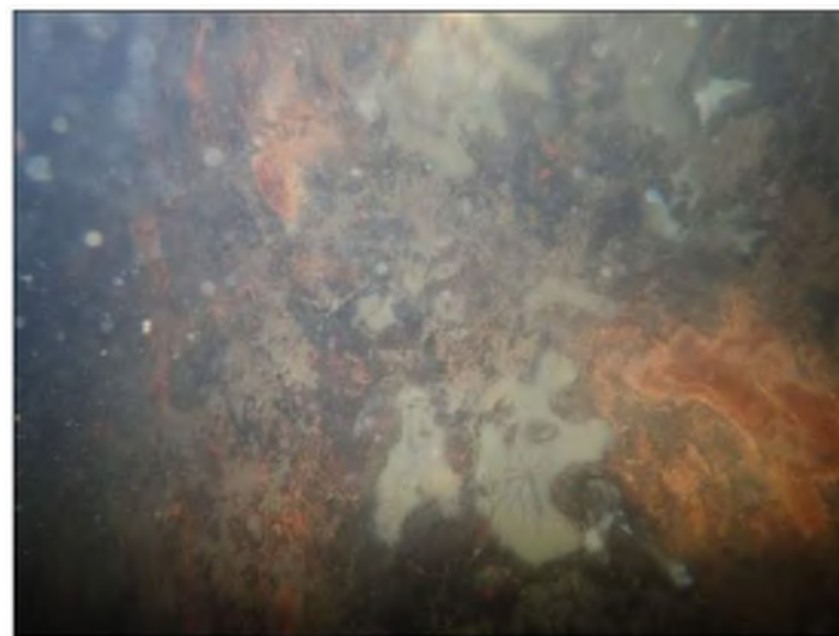
Photo 05: Quay Wall Substructure Typical condition of steel sheet pile cells at mid-depth
