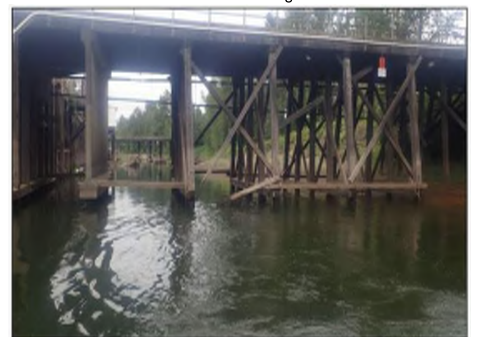
Photo 06: Berth 311 Trestles East Trestle Broken cross-bracing
