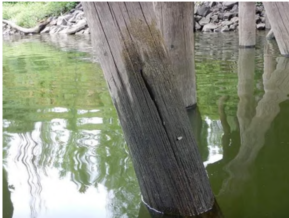
Photo 04: U.S. Navy Pier Dolphins Typical condition of timber batter pile Source: AME 2019 Report
