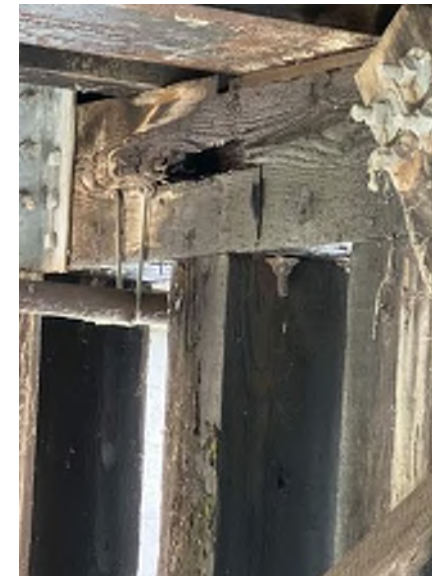
Photo 08: Berth 311 Main Pier Pile Cap at Bent 2 Loss of section on pile cap Moata ID: 74406
