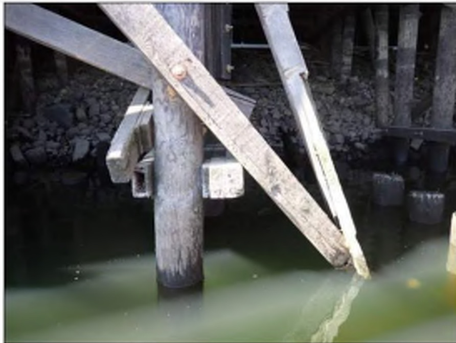
Photo 08: Lagoon Wharf Substructure Typical timber decay in walers and cross-bracing
