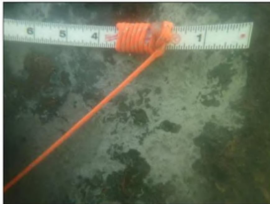
Photo 03: East, West, and Demo Piers Substructure Typical cleaned surface of steel piles at mid-depth
