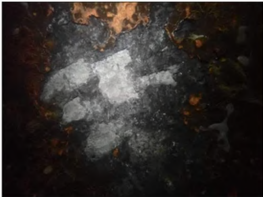
Photo 04: Pier A Substructure Typical cleaned steel below waterline
