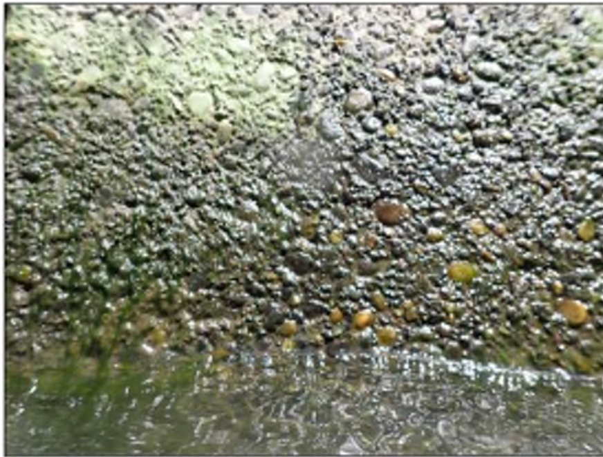
Photo 01: East, West, and Demo Piers Substructure Typical condition of concrete bearing piles at waterline
