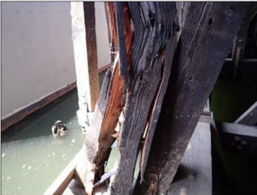
Photo 04: Berth 311 Substructure Piles I and J Bent 23 Broken piles
