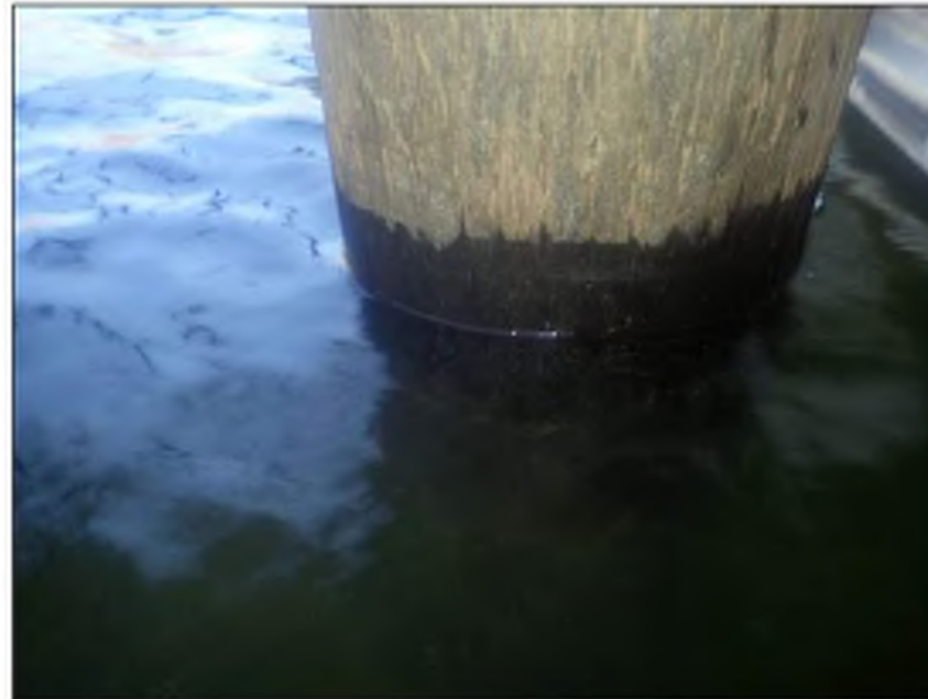
Photo 02: Dredge Base Overview Typical condition of timber piles at waterline
