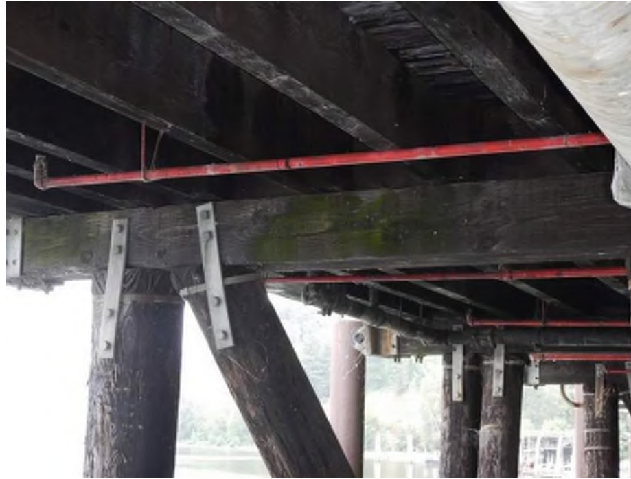
Photo 02: U.S. Navy Pier Substructure Typical condition of timber pile cap Source: AME 2019 Report
