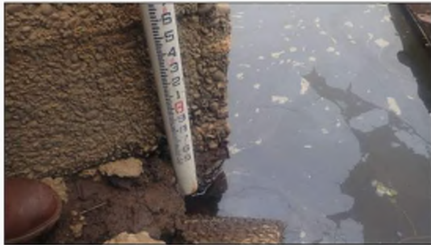
Photo 01: City Stormwater Outfall M2 Wingwalls Typical condition of concrete at waterline
