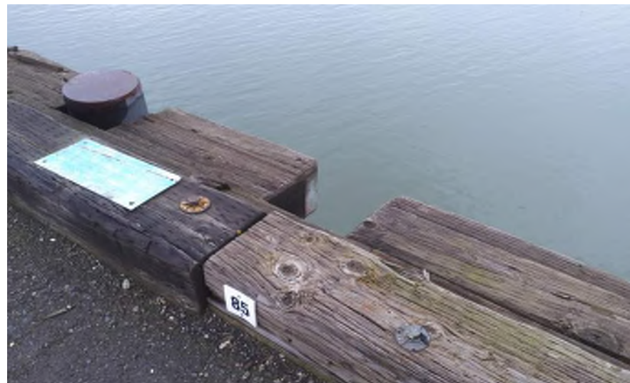
Photo 03: Lagoon Wharf Fender System Adjacent to Bent 85 Missing fender pile Moata ID: 73552
