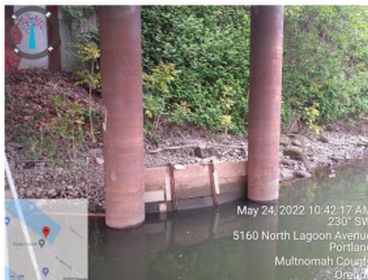
Photo 04: Wind Tunnel Substructure Piles A and B, Bent 1 Typical condition of piles above water Moata ID: Not Applicable
