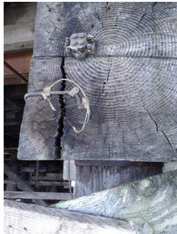
Photo 07: Lagoon Wharf Substructure Adjacent to Bent 72 Split on the pile cap Moata ID: 73610
