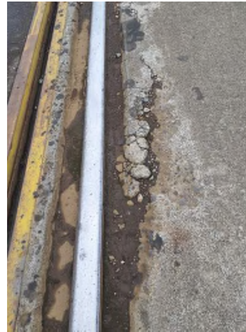
Photo 02: Pier D Superstructure Bent 50 between Piles E and G Concrete spalls around crane rail Moata ID: 73693
