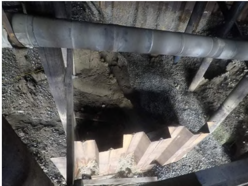
Photo 03: City Stormwater Outfall S1 Embankment erosion behind and adjacent to headwall
