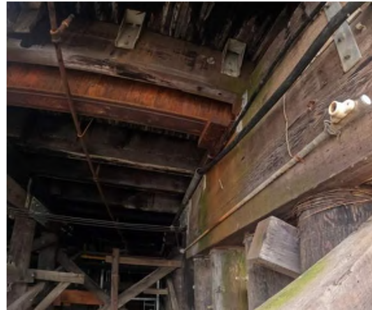
Photo 06: Lagoon Wharf Substructure Typical condition of crane rail Moata ID: 73587
