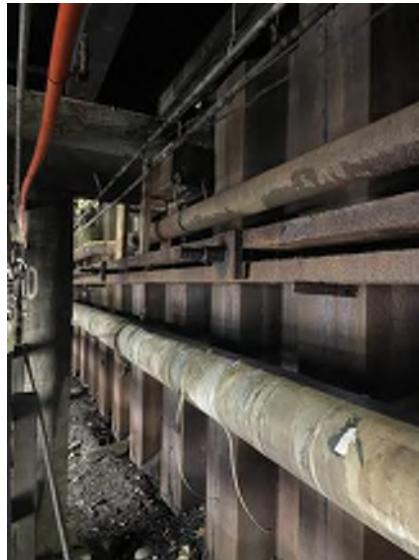
Photo 16: Lagoon Wharf Substructure Steel Sheet Piles between Bents 85 and 92 Typical condition of walers Moata ID: Not Applicable
