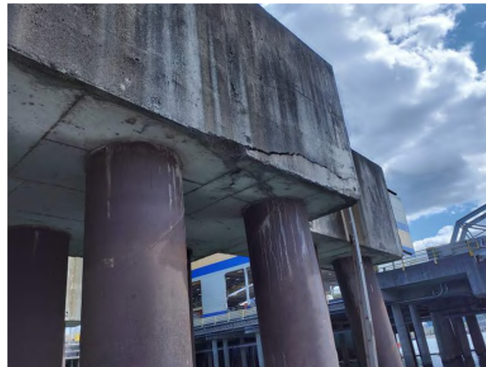
Photo 04: Demo Pier Substructure Pile Cap at Bents 7 Pile C1 Closed spall at corner of the pile cap Moata ID: 74979
