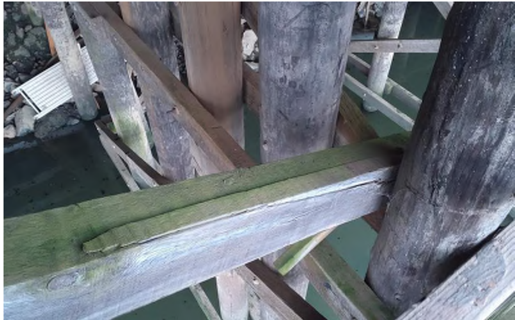
Photo 13: Lagoon Wharf Substructure Adjacent to Bent 16 Split on the timber cross-bracing Moata ID: 73580
