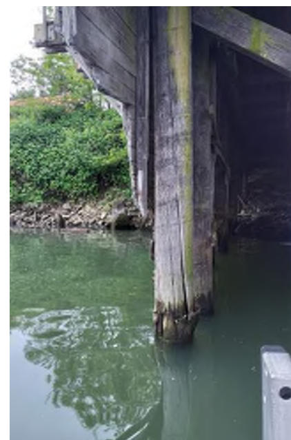
Photo 21: Lagoon Wharf Substructure Adjacent to Pile A Bent 135 Split on the timber pile Moata ID: 74984
