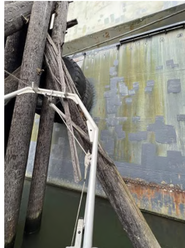
Photo 05: Lay Berth 306 Dolphin Dolphin D3 Partially broken pile Moata ID: 75036
