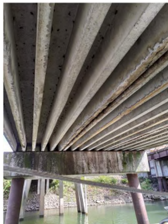
Photo 03: West Pier Substructure Concrete Girders between Bent 3 to Bent 4 Concrete spalls exposing reinforcement due to corrosion Moata ID: 74980
