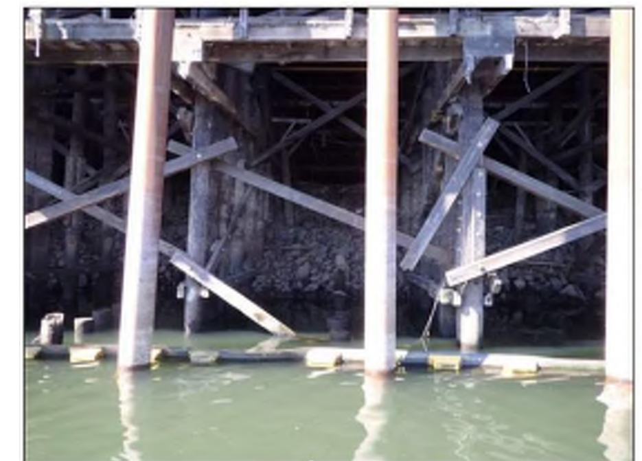
Photo 06: Lagoon Wharf Substructure Typical damaged cross-bracing
