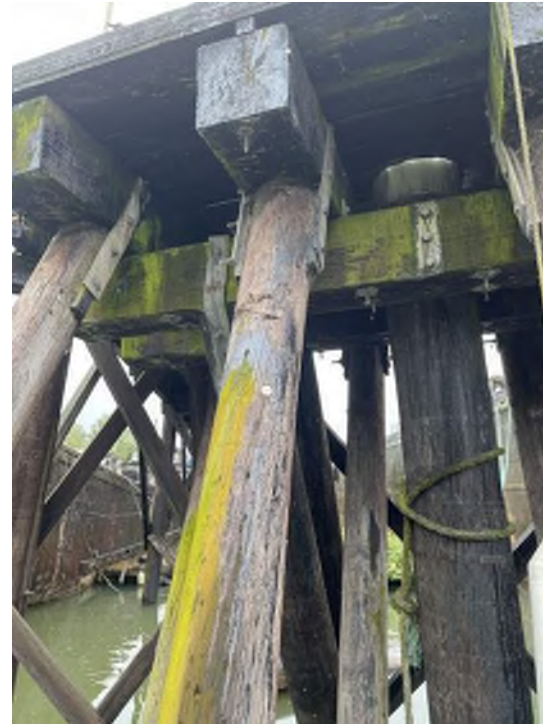
Photo 02: Berth 311 Dolphin West Dolphin Typical condition of piles Moata ID: 74374
