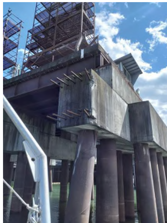
Photo 03: Demo Pier Substructure Pile Cap at Bents 7 Pile J Impact spalls at corner of the pile cap Moata ID: 74979
