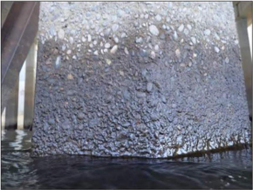
Photo 02: Pier D Substructure Typical condition of concrete piles at waterline
