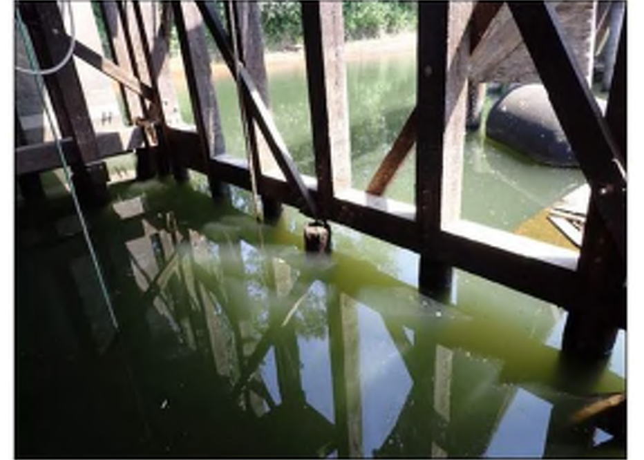
Photo 03: Berth 311 Substructure Pile 4 Bent 31 Pile non-bearing
