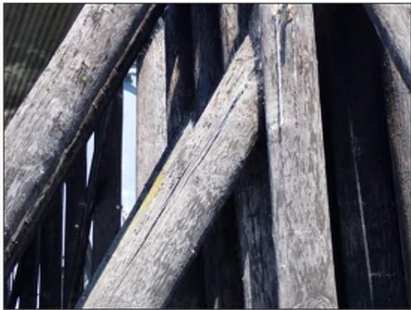
Photo 04: Lay Berths 306 & 307 Dolphins Dolphin D4 pile 6 Internal decay in pile
