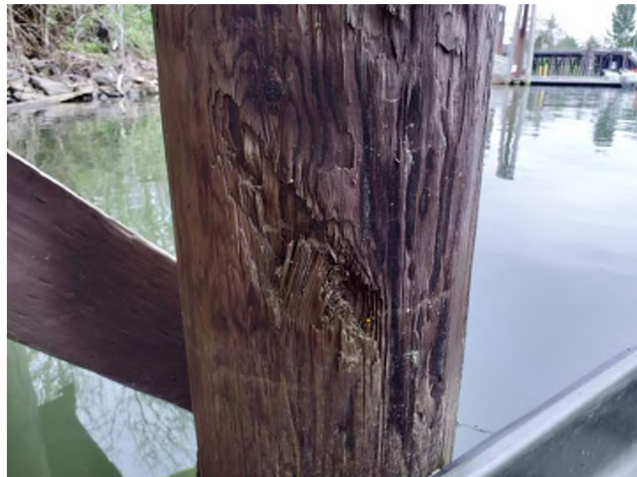
Photo 04: U.S. Coast Guard Dock and Pier Substructure Pile D Bent 6 Loss of section on the pile Moata ID: 74998
