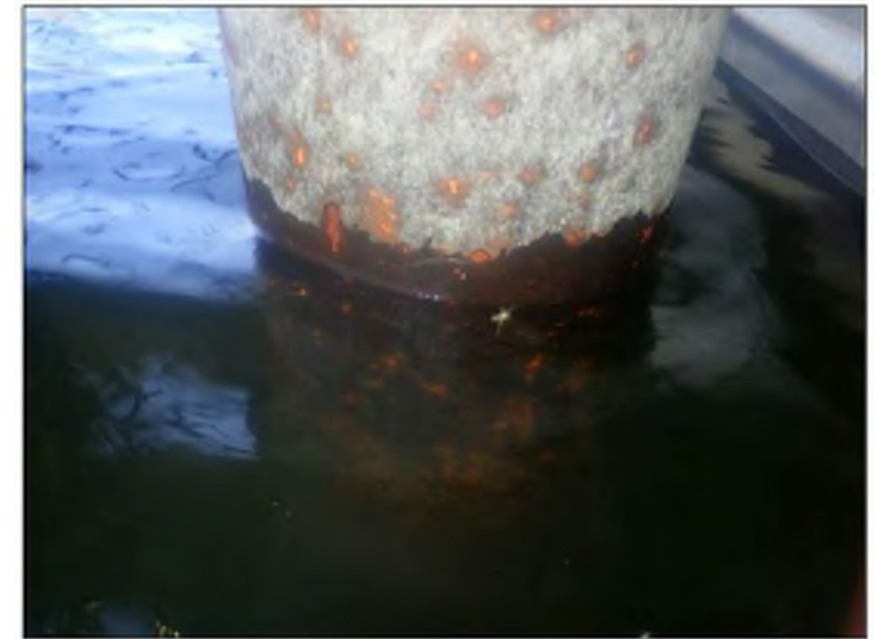
Photo 03: Dredge Base Overview Typical condition of steel piles at waterline
