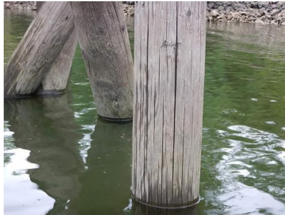
Photo 05: U.S. Navy Pier Substructure Typical condition of timber pile Source: AME 2019 Report
