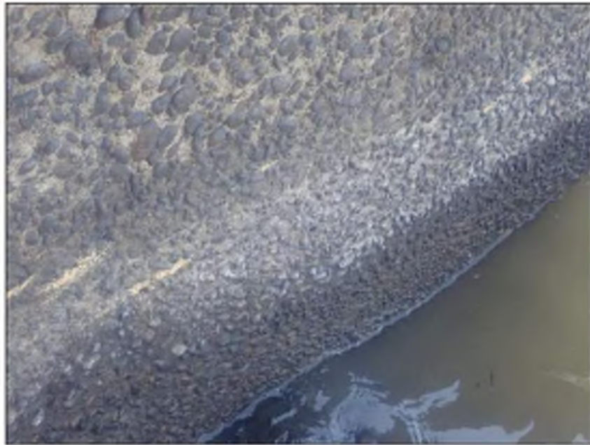
Photo 01: City Stormwater Outfall M1 Typical abrasion on concrete
