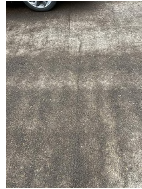
Photo 03: Berth 311 Trestle West Trestle Cracks on the concrete deck Moata ID: 74378
