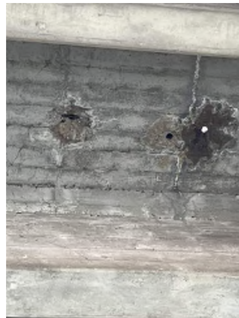
Photo 04: Pier C Superstructure Underside of Concrete Deck Between Bents 4 and 5 Concrete open spall exposing reinforcement Moata ID: 75112
