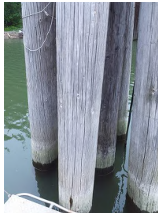
Photo 05: U.S. Coast Guard Dock and Pier Dolphin Dolphin D11 Typical condition of Dolphins (Main Pier) Moata ID: 75009
