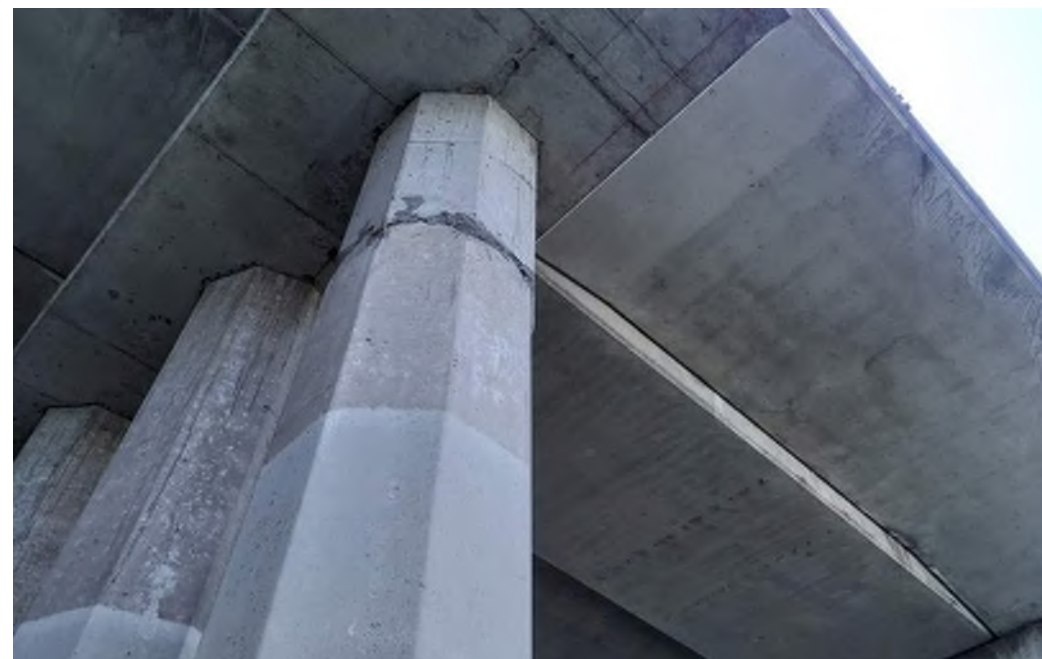
Photo 05: Pier D Substructure Pile K at Bent 43 Concrete spall around full diameter of the pile Moata ID: 74344
