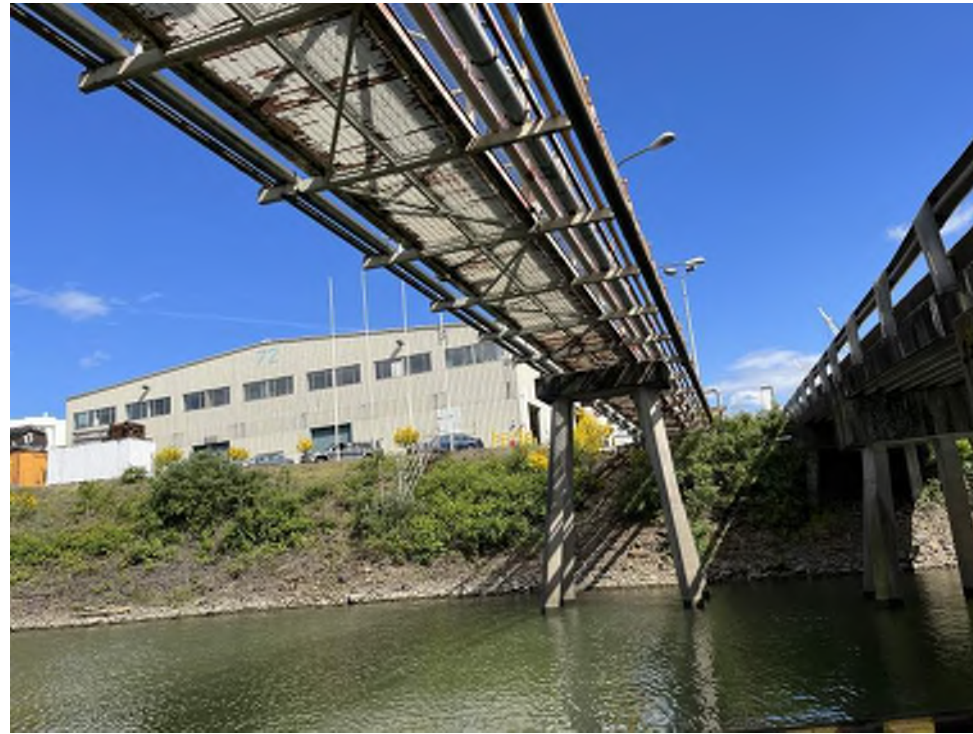
Photo 01: East Pier Substructure Substructure between Bent 1 and Bent 2 Typical configuration of substructure Moata ID: Not Applicable
