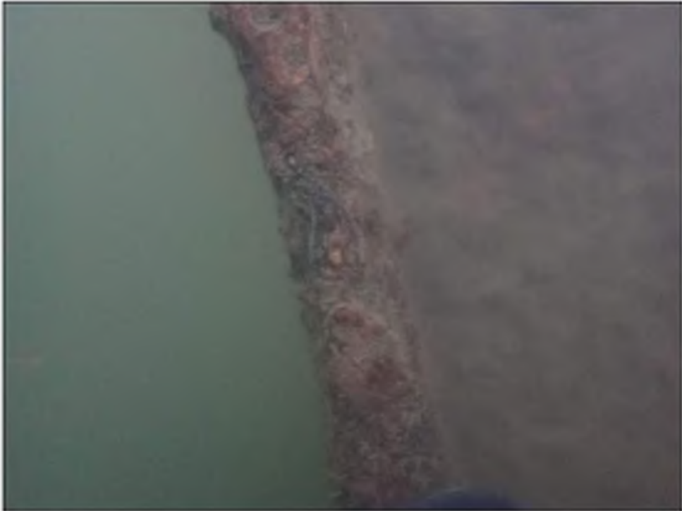
Photo 04: Pier D Substructure Typical condition of steel batter piles flange below waterline
