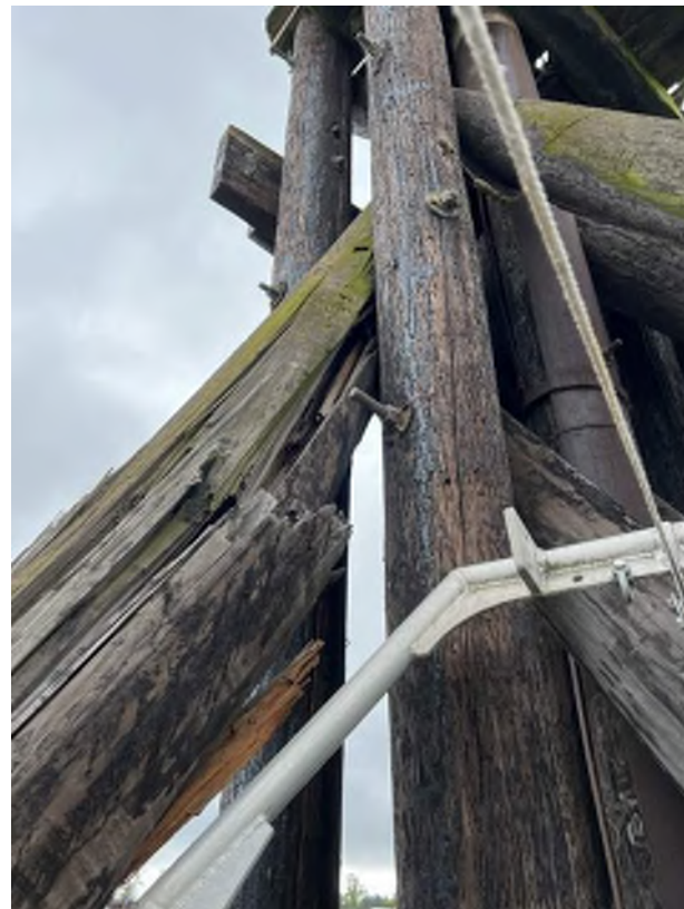
Photo 04: Lay Berth 306 Dolphin Dolphin D1 Partially broken pile Moata ID: 75029
