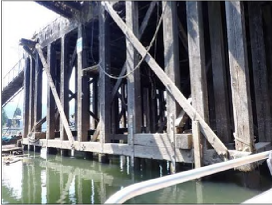
Photo 01: Berth 311 Substructure Typical substructure configuration, looking west
