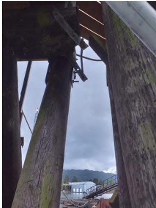
Photo 01: Berth 311 Dolphin East Dolphin Loss of connection between batter pile and deck Moata ID: 74395
