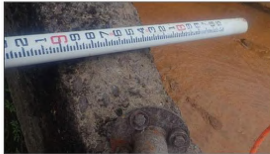
Photo 02: City Stormwater Outfall M2 Wingwalls North Wingwall Spall on north waingwall
