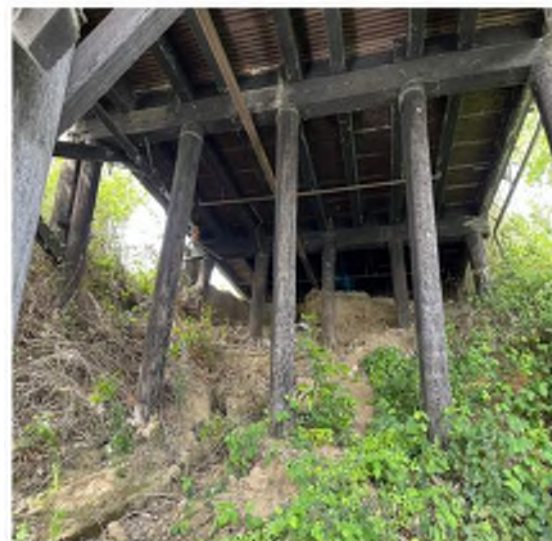
Photo 04: Berth 311 Trestle West Trestle Typical condition of piles Moata ID: Not Applicable
