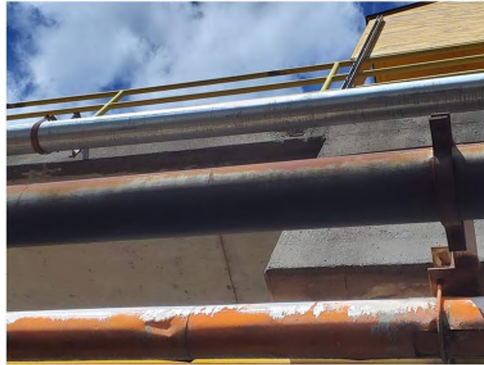
Photo 02: East Pier Superstructure Deck between Bents 2 and 3 Concrete spall exposing reinforcement Moata ID: 74981
