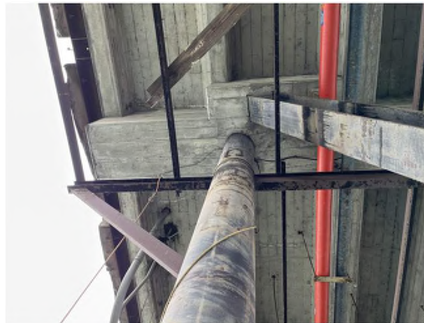
Photo 05: Pier C Superstructure Concrete Pile Cap at Pile C Bent 40 Concrete closed spall on the bottom of the pile cap Moata ID: 75133
