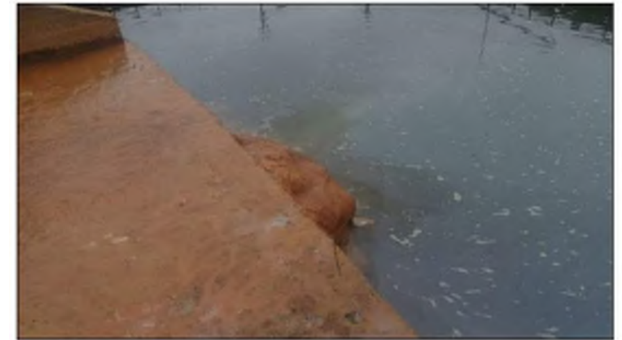
Photo 03: City Stormwater Outfall M2 Base Material build-up at base of outfall
